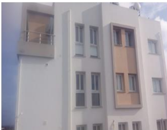
Fig. 14a showing the openings on the south facade
